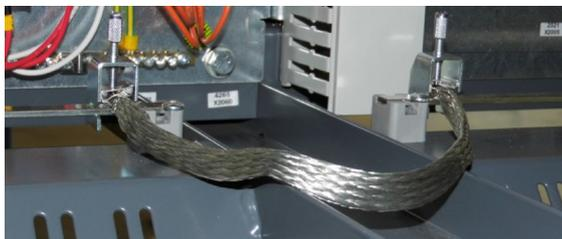
Figure 1: Mounting rail for cable braid bonding.
